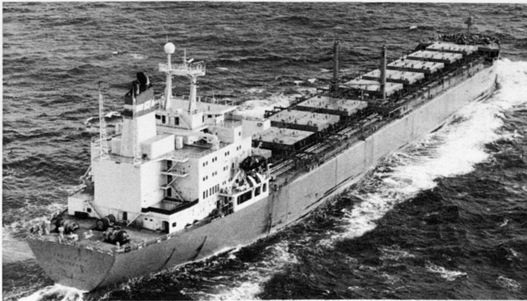
FIGURE 3. The ship Earth station, which enables a ship to communicate with other ships or with shore-based subscribers, consists of equipment both above and below deck. Above deck is a parabolic antenna on a stabilized platform covered in a radome. The radome on the bulk carrier Ambia Fair can be seen here as a white, distinctive mushroom shape mounted on a pedestal above the bridge. (Photograph by Skyfotos.)
